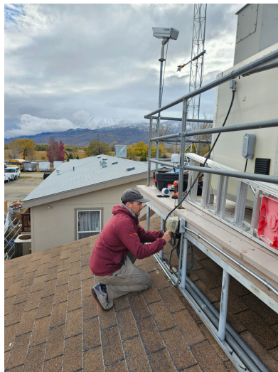
Picture description: GBUAPCD and EMO staff installing the particles sensor at the BPT Air Monitoring Station
