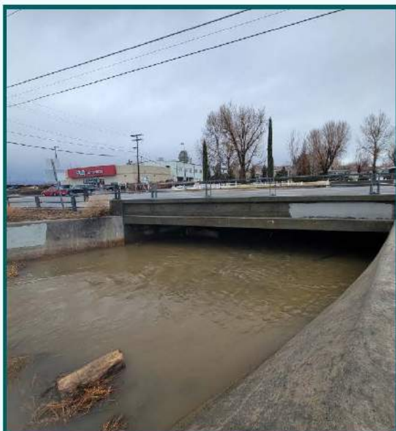
Figure 1: Downstream view of SW-2 Bishop Creek site before the water leaves the Reservation as it flows beneath highway 395. Photo taken 01-10-2023
